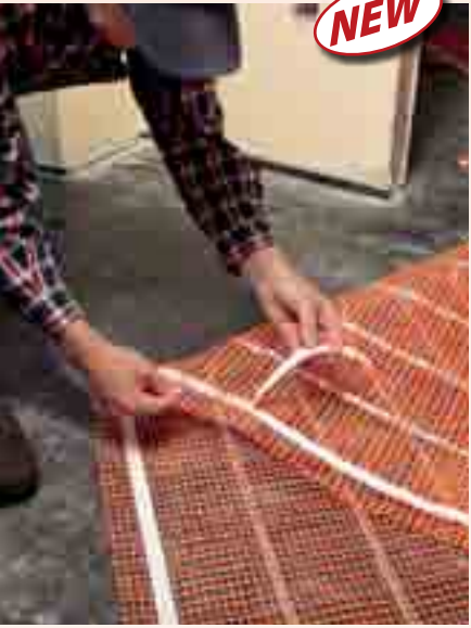
Roll out mat and secure to the floor using new adhesive strips.
