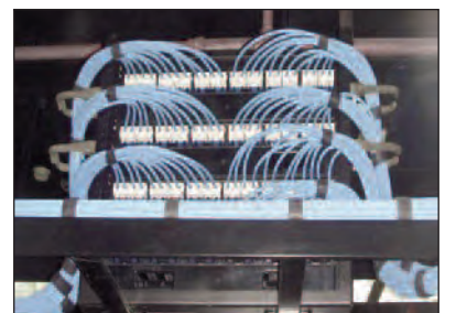
PatchRack with D-Rings installed on CPI Cable Runway above CPI TeraFrame® Cabinet.
