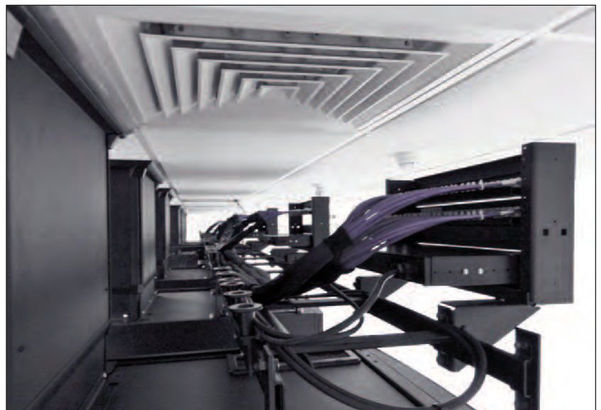
Rear view of PatchRack installed on CPI Cable Runway above CPI TeraFrame® Cabinet.
