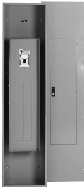
Main Circuit Breaker Commercial
