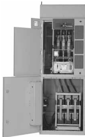
AMPGARD IT. Soft Start (Doors Open)
