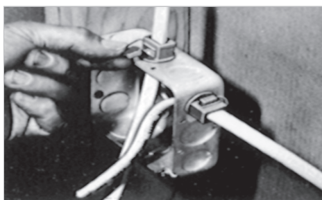
Snap captive locking wedge into fitting's cavity
