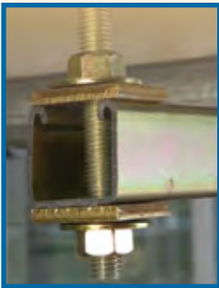
Standard method using nuts and washers
