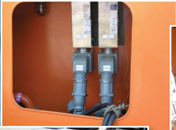
200A MaxGard® inlets with disconnects
