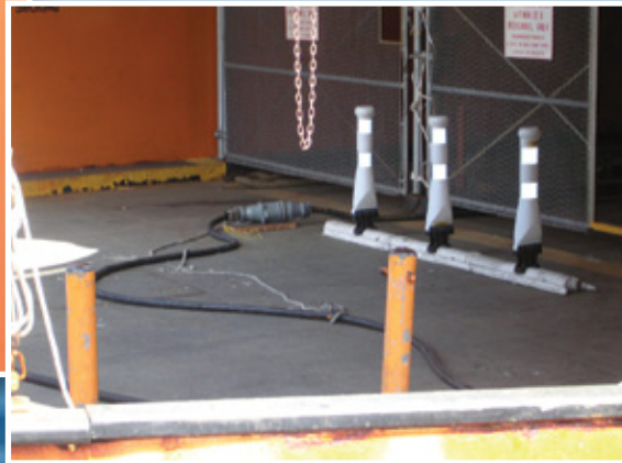
200A MaxGard® connections on ferry deck
