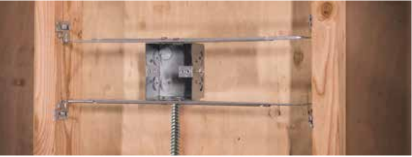
Step 3: Cut channel and mount channel to studs or perforated metal sheets (provided) with screws
