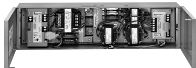
Voltage Module Interior View
