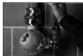
5. Install hub on enclosure
