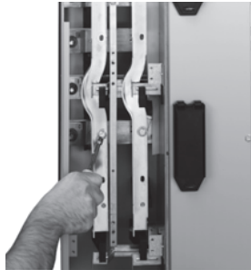
Field Phase Balancing
