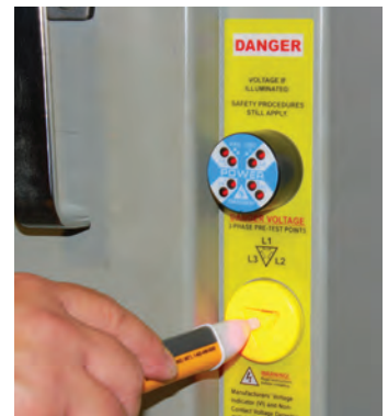
Fig. 8 Panel Mounted Indicators
