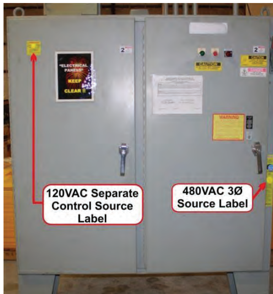
Fig.1 Voltage Source Labeling
