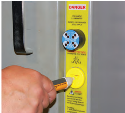
Fig. 9 Verifying proper operation of the NCVD
