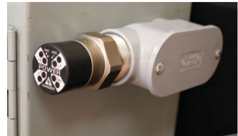
1 1/2 conduit vertical with R-3W
