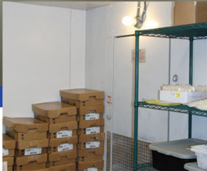
Safety coated incandescent heat lamps in food service and globe covering an A19 in a walk-in cooler.
