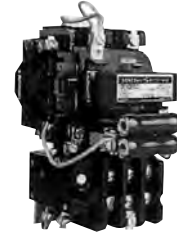
Space Heater Installed on Typical NEMA Size 1 Starter
