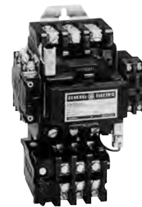
Typical Size 2 Starter with CR305X Control Amplifier Mounted on Right
