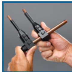
4. Slide connector/insulator assemblies onto rod.
