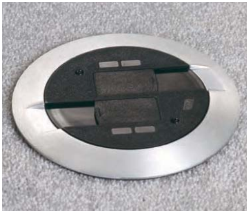
RC9AMD Series Poke-Thru Device (RC9AMDTCAL) installed in a carpeted floor.
