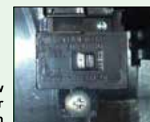
Pick-A-Flow Speed Selector Switch
