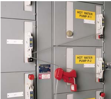
The Cable Lockout Device enables you to lock out several disconnects in various energy distribution centers.
