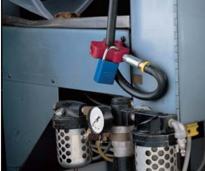
Using T&B's Pneumatic Quick-Disconnect Lockout to isolate pneumatic energy provides worker safety in lock out situations.
