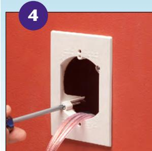
**4** Tighten screws. Mounting wings hold mounting bracket securely against drywall – No wobble once it is installed!
