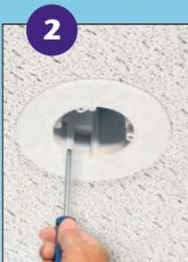
2 Install CAM-BOX™ kit. Rotate to desired position. Tighten mounting wing screws.
