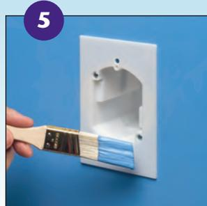
**5** If desired, paint front surface to match wall. Install device.
