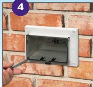
**4** Attach IN BOX with screws provided. Install wiring device per manufacturer's instructions, Local and National Electrical Codes.
