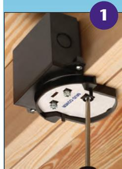
**1.** Position box alongside joist. Tighten center screw, mounting box to joist.
