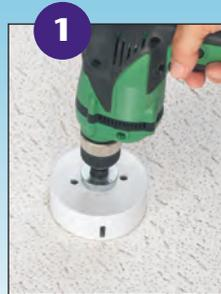
**1** Cut hole in a ceiling grid with 4" hole saw. 4-1/2" for steel.
