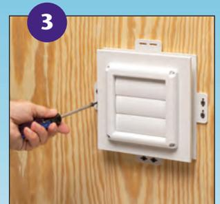
3 Use screws to mount dryer vent to substrate through flanges.
