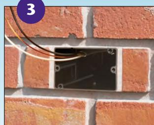
3 RAYS BOX installed flush with masonry surface, ready for installation of device or fixture.
