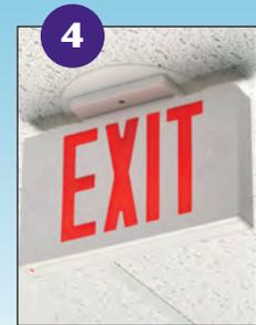
**To Complete:** Using the appropriate KO (1/2" or 3/4") install NM94 cable connector (supplied) and pull cable. Install fixture per manufacturer's instructions.
