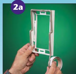
2a Apply caulk around edges of back of adapter. Press onto siding.
