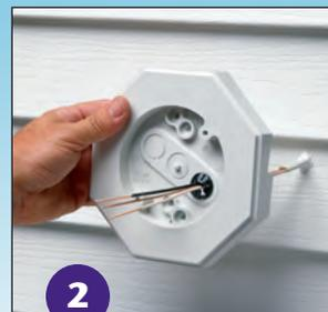
2 Remove knockout from electrical box and insert cable connector. Push cable through connector and position mounting block onto siding.
