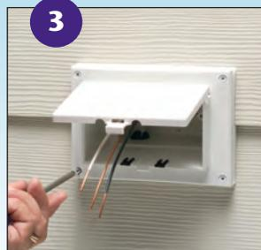
Apply caulk to reverse side of IN BOX flange (see page J-14, step 3a). Install NM cable connector and wire, then attach with provided long screws. Trim excess caulk as needed.
