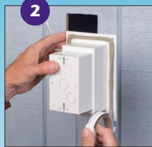
2 Apply the supplied caulk around back edges of flange. Install NM cable connector and wire, then press onto surface.
