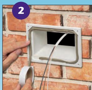
**2** When ready to complete... apply supplied caulk as shown and press around edges of adapter sleeve.
