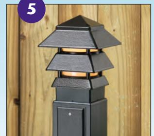
6 Install pagoda light to post with locknut inside the top of the post. Wire fixture.
