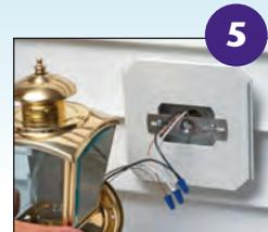
5. Connect wires and install fixture per manufacturer's instructions.
