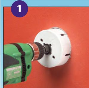
**1** Determine mounting bracket location. Cut opening with a hole saw; 3.5" for single-gang LV1RP, 4.5" for the 2-gang LV2RP.
