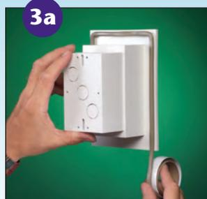
3a Apply caulk to reverse side of IN BOX flange.
