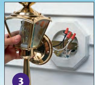
3 Secure mounting block with provided screws. Install fixture per manufacturer's instructions.
