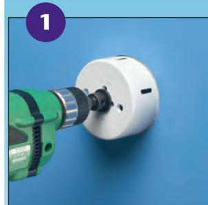
**1** Determine box location. Cut opening with a hole saw; 3.5" for single-gang **FD1RP**, 4.5" for the 2-gang **FD2RP**.
