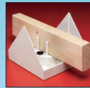
Cut a 2x4 approximately 14" long to span the pitched rafters.
