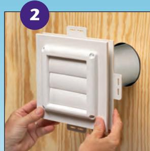
2 Insert vent tube into opening.
