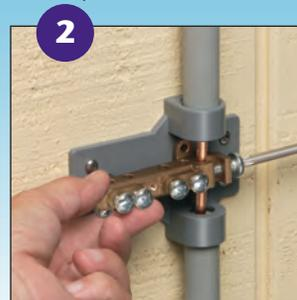
Insert grounding electrode conductor into the lay in lug. Tighten screw.
