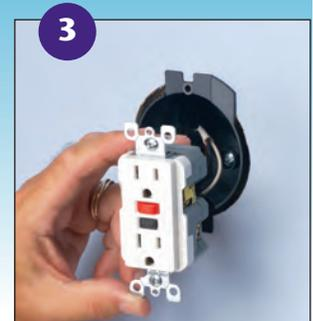
3 Install device (GFCI shown) and provided maxi-size cover plate.
