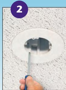
**2** Install CAM-LIGHT™ box. Rotate to desired position. Tighten mounting wing screws.
