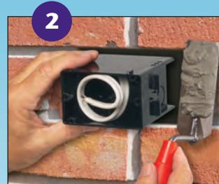
2 Mortar in box. Built-in tabs set in the mortar hold the box securely in place.
