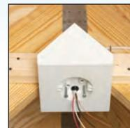
Push the cable through the installed cable connector in the electrical box.
