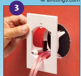
**3** Insert mounting bracket into the opening. Rotate as necessary to level. Shown with single-gang LV1RP.
