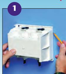
Using box, without trim plate as a template, mark location. Cut hole.
