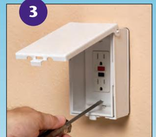
**3** Install plate and the installation is done!
