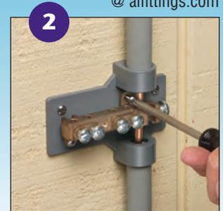
Insert grounding electrode conductor into the lay in lug. Tighten screw.
