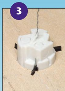
3 Add drop wire to loop. Attach to framing member above.
