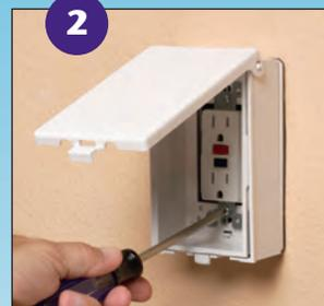
**2** Install wiring device per manufacturer's instructions, Local and National Electrical Codes using the pre-drilled holes in base.
