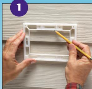
Using the siding profile adapter plate as a template, cut hole in existing siding. Pull wiring.
