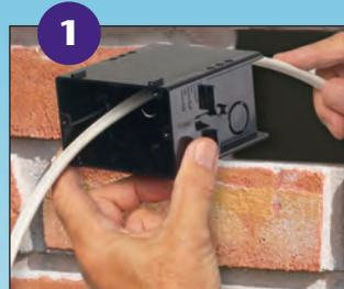
1 Pull cable through installed NM cable connector. (NM94 cable connector included with each box.)
