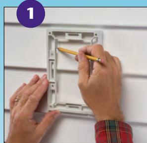
1 Using the siding profile adapter plate as a template, cut hole in existing siding. Pull wiring.
