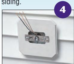
4. Place siding block over box section (8081 shown).
