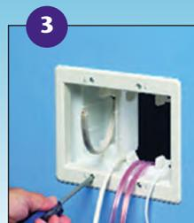
Tighten mounting wing screws to pull the box securely against the wall board. See Photo B.
