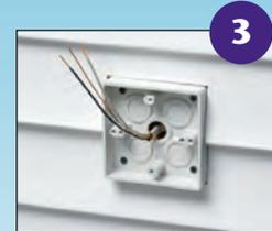
3. Mount box section to substrate. Caulk as required.
