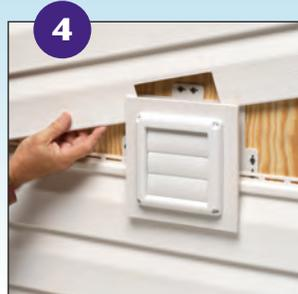
4 Install siding. Overhang on vent flange hides cut ends of siding.
