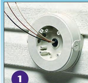
1 Pull wire and attach box to siding surface.
