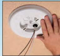
**2.** Using the #8 x 1-1/2" wood screws provided, mount the MB8 to the joist (through the ceiling).
