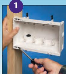
1 Mount box to stud. Use tabs for proper positioning of box for 1/2" wall finish. See Photo A.
