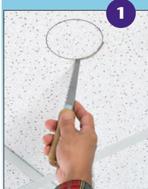
1. Cut a 4-1/16" diameter hole in the center of a 24" ceiling tile. Place box over hole. Snap plastic ends of support bar over the ceiling grid.
