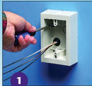
1 Pull wire and attach box to flat surface.
