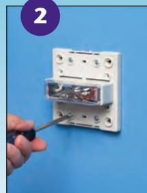
Install fire alarm (or other device) through the screw holes in the box.
