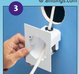
**3** Push cable through connector. Insert box into the opening. Shown with single-gang **FD1RP**.
