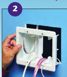
Attach trim plate to box. See Photo B. Pull wire/cables. Install box assembly in opening.
