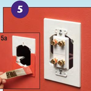
**5** If desired, paint front surface to match wall (photo 5a). Install low voltage device.
