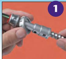
1 Snap cable into fitting until it stops. Rotate cable clockwise to lock in place.
