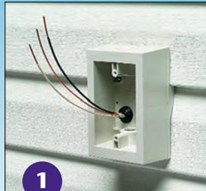
1 Pull wire and attach box to siding surface.
