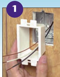
**1** Pull wires through, then press the BE1 firmly into the electrical box.
