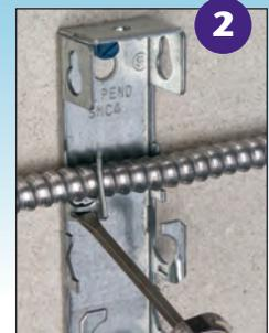
Bend tab over cable, locking it securely in place.
