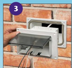
**3** Install the supplied NM cable connector and wire. Insert the clean IN BOX into the sleeve.
