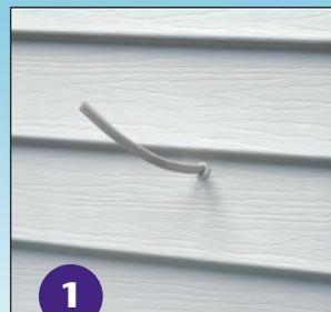
1 Select location for light fixture and caulk opening around cable.
