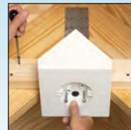
Position the 2x4 with the FB900 attached to the angled rafters, keeping bottom of box level, and the short sides of the box touching the angled rafters. Nail or screw the assembly, spanning both angled rafters.
