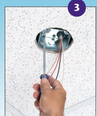
3. Pull cable through installed NM cable connector and remove captive screws for fan/fixture bracket installation.
