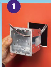
Determine position of device. Cut hole. Pull wire(s) through appropriate knockout (connector). Install box in opening. **FSR404S** shown.
