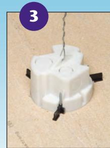
**3** Add drop wire to loop. Attach to framing member above.
