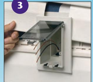
3 Install siding, inserting the cut ends of the siding under the outer flange of the IN BOX.
