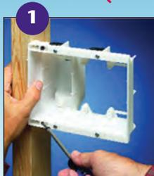
Attach box to stud. Use tabs for proper positioning of box depth. See 2.
