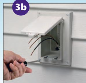
3b Install NM cable connector and wire, then attach with provided long screws. Trim excess caulk as needed. Install wiring device per manufacturer's instructions, Local and National Electrical Codes.
