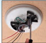
**3.** Install the fixture or fan mounting bar (provided with the fixture or fan) directly to the joist with the (2) #10 x 3" wood screws and lock washers provided. Wire the fixture or fan following the instructions included with the product.
