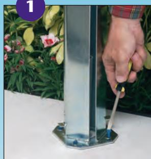
1 Metal support post attaches easily to surface.
