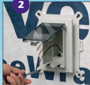
2 Install NM cable connector and wire, attach IN BOX to substrate.
