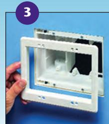
Attach paintable trim plate with screws provided. See Photo B.
