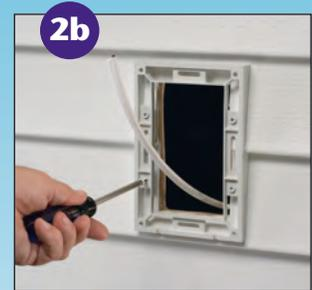
2b Attach adapter to siding with provided short screws. Trim excess caulk as needed.
