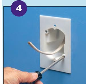
**4** Level the box. Tighten the mounting "wing" screws to pull the box snug against the drywall.
