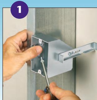
Determine size of stud. Bracket is preset for a 2x6 stud with 1/2" wall finish thickness. Attach box to wood or metal stud with the captive screws inside the box. **F101S** shown.
