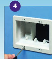
Tighten mounting wing screws to pull the box securely against the wall board. See Photo B.
