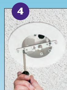
4 Add bracket to the box using screws provided.
