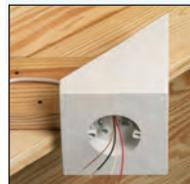
Push the cable through the installed cable connector in the electrical box.
