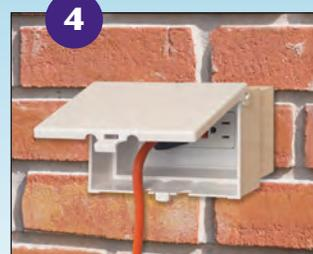
4 Outlet installed. Caulk as required around the outdoor cover. Shown with Arlington's IN AND OUT™ Cover. See page J-25.
