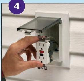
4 Install wiring device per manufacturer's instructions, Local and National Electrical Codes.
