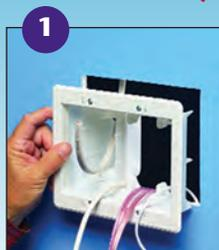
1 Using box as a template (without trim plate), mark location. Cut drywall. Attach trim plate to box. See **Photo B**. Install box assembly in opening.
