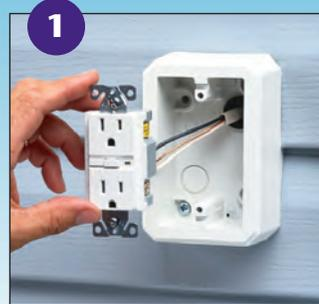
Remove KO from FS Box and insert NM cable connector. Push cable through connector and position box onto siding.
