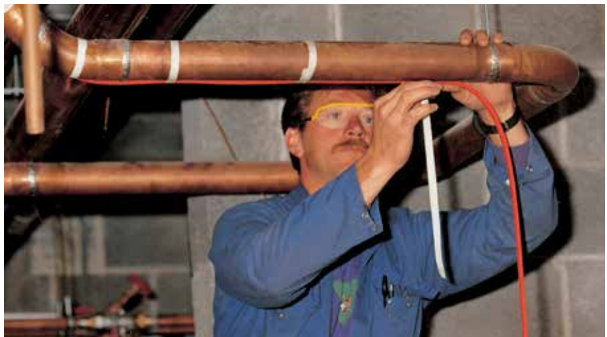
The lengths of pipe correspond to the lengths of heating cable needed.
