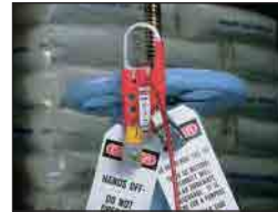
Lockout gate valves
