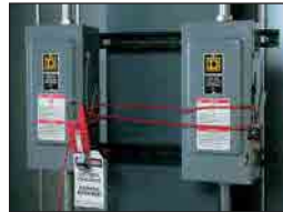
Lockout single or multiple electrical disconnects
