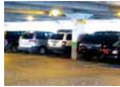
Garage Lighters provide safety and security in parking garages
