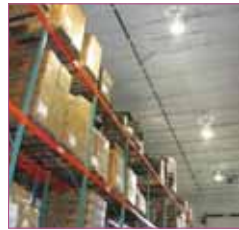
Hi Bay fixtures are a popular lighting source in warehouses
