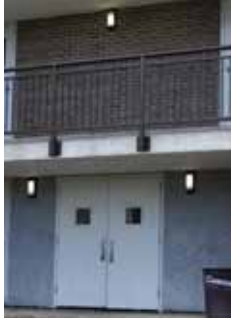
This college dorm's rear entrance stays safely lit with RAB's VAN 6 Vandalproof fixtures.
