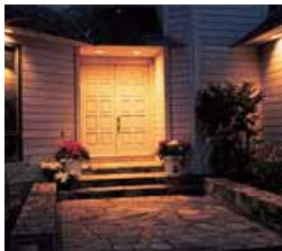
Smart Box controls 500 watts of front door lighting. (Hint: Look on the wall to the left of the door.)
