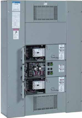
Elevator Control Panelboard
