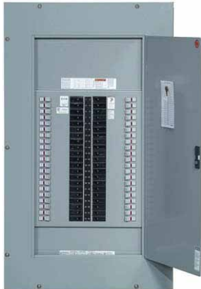
Type PRL1a Panelboard
