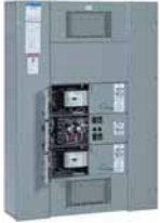
Elevator Control Panelboard
