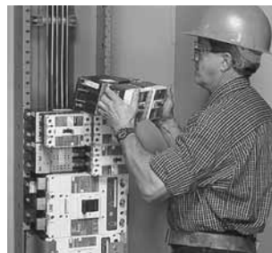
Panelboard Installation
