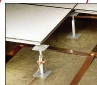
Signal Reference Grid (SRG)
