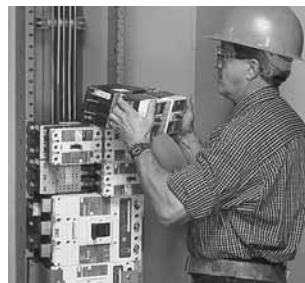
Panelboard Installation
