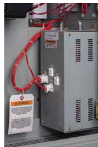
Multi-Tap Control Power Transformer
