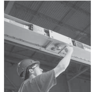
Typical Busway Installation (Torque Indicating Bolt)
