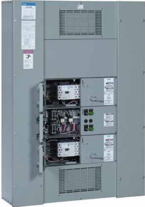
Elevator Control Panelboard
