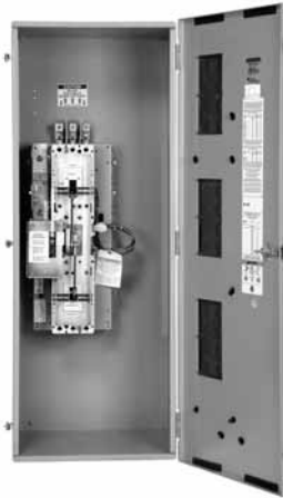
Manual Transfer Switch Shown Without Deadfront
