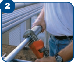
With a wrench, tighten the gland nut to compress the Teflon® packing, creating a raintight seal around the conduit.
