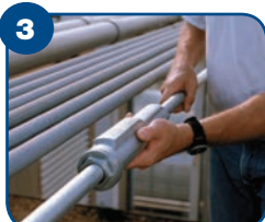
Thread the next length of conduit into the other end of the fitting and tighten. You're done!
