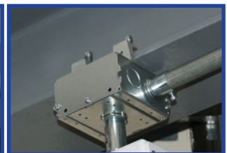
(4) Attach side plate with screws to finish installation
