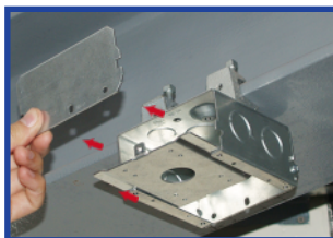
(1) Install EALB with side plate and cover plate REMOVED
