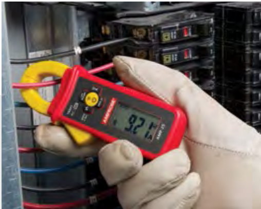
Troubleshoot electrical systems and measure AC/DC load current on exposed wires in a breaker panel.
