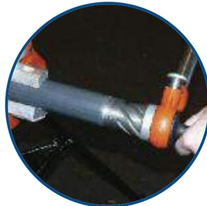
Ream the conduit with approved reamers. Spiral and straight-style reamers are both acceptable.
