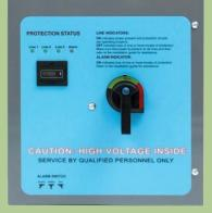
The PG4000 Series is a hardwired suppression device (installed in parallel) and recommended for all ANSI/IEEE Category locations.
