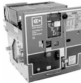
Power Breaker Replacement
