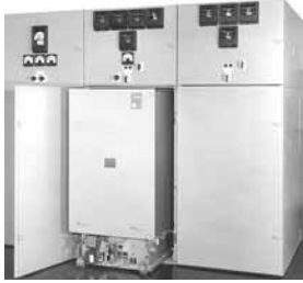
Medium Voltage Switchgear Assembly (Type DHP with Drawout Breaker)
