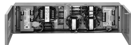
Voltage Module Interior View
