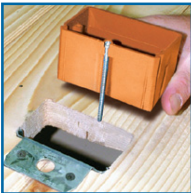
Install clip over subfloor.
