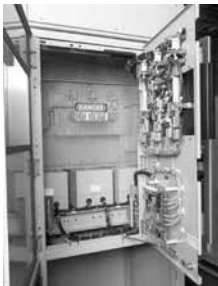
Mark V Field Controller
