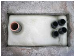
Sticks brought into transformer through visible rodent hole next to conduit
