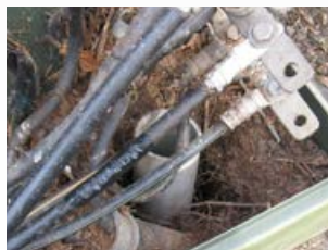
Sticks brought into transformer through visible rodent hole next to conduit
