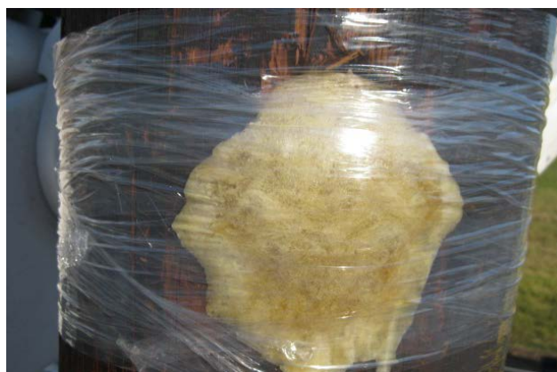
Woodpecker damage repaired with UPR™ Pole Repair
