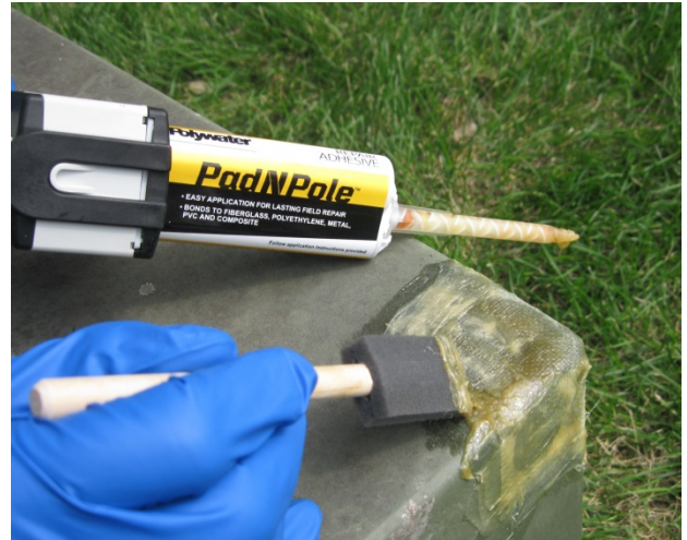
Fiberglass cloth saturated with the high-strength, two-part resin makes the permanent PowerPatch® Pad N Pole™ Repair.
