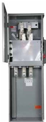
Main Fusible Switch with Utility Pull Box
