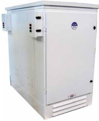
Double Panel Substation
