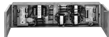
Voltage Module Interior View
