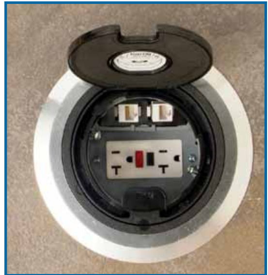
Power and Communications
