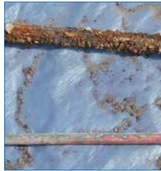
Excavated after 12 years.
