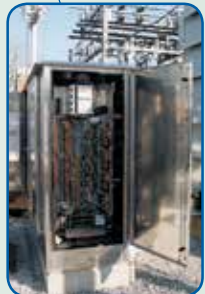
Power and Control Surge Protection for SCADA and Power Connections
