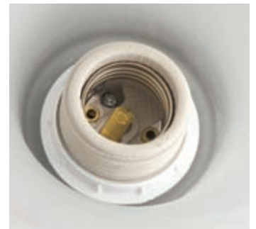
Shade secured in place.
