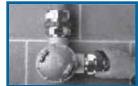
6. Insert cable and tighten red union
