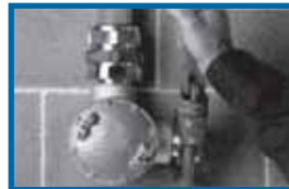
5. Install hub on enclosure
