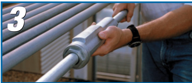
Thread the next length of conduit into the other end of the fitting and tighten. You're done!
