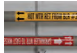
Pipe & Valve ID
