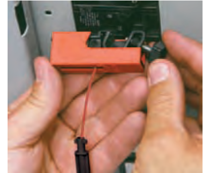
2 Attach the lockout device to the breaker and snap into locked position.
