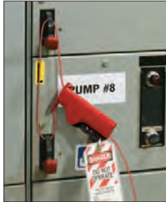
Lockout multiple control points with a single device.
