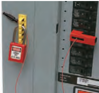
3 Pass plastic key through lock rail and attach lock, preventing key from sliding down cable and opening lockout device.
