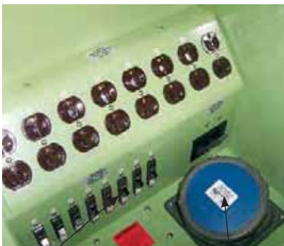
Circuit Breakers (Prewired to Receptacles)
