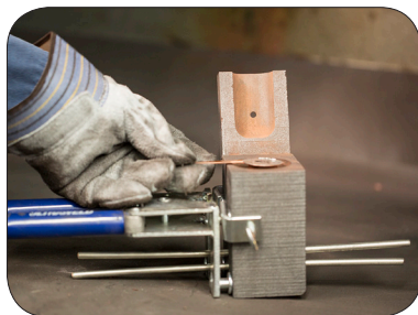
Step 2: Place conductors and UltraShot cartridge into mold.
