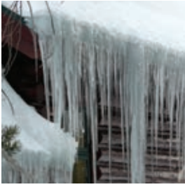
Unprotected roof and gutters
