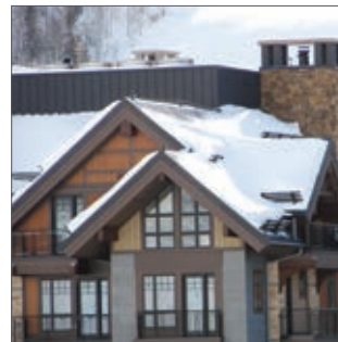
Roof & Gutter De-Icing
