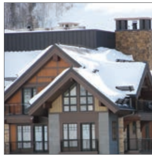
Roof & Gutter De-Icing
