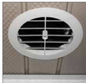
EZ Soffit Vent installed
