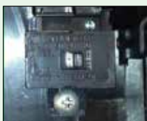
Pick-A-Flow Speed Selector Switch
