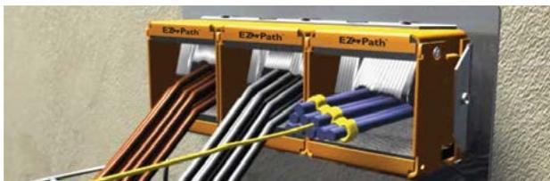
Only the EZ-Path System requires no unsealing, resealing or adjustment of any kind. Pulling lines can be left in place and cables can be remotely pulled through multiple barriers. So no direct access is required other than the beginning and end of the pull. No other product offers this feature.
