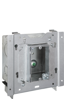
T5 Box Installed
