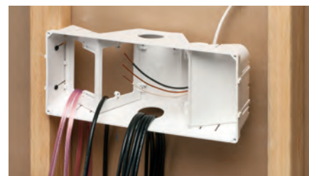
2 Pull power and low voltage wire. After installing the wall, continue with retrofit steps 3 and 4 (above).
