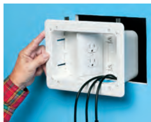
1 Cut Top hole in wall for the TV Box. Cut Lower hole directly below the top hole, close to an existing outlet.
