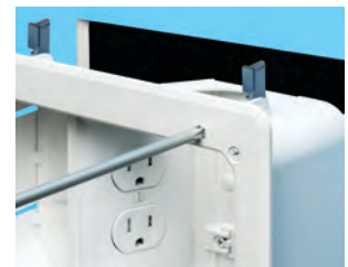
3 Place box in Top hole. Feed low voltage cables for TV through opening in box. Tighten mounting wing screws to secure box to wall. (continue with Lower Box installation on facing page)
