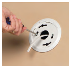
3 Install mounting plate per manufacturer's instructions
