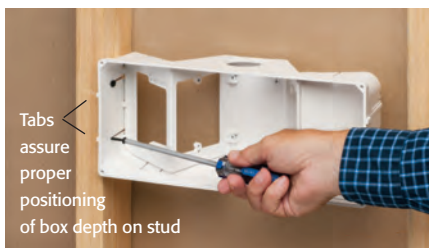
1 Attach box to stud through slotted holes.
