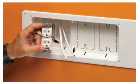
3 Install power and low voltage wiring devices.
