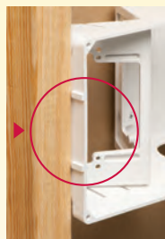
3 Install enclosure assembly to wall with outer screws.
