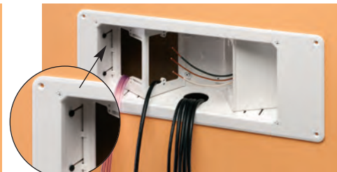
2 Attach assembled enclosure w/ trim ring to stud through slotted holes in the side walls.
